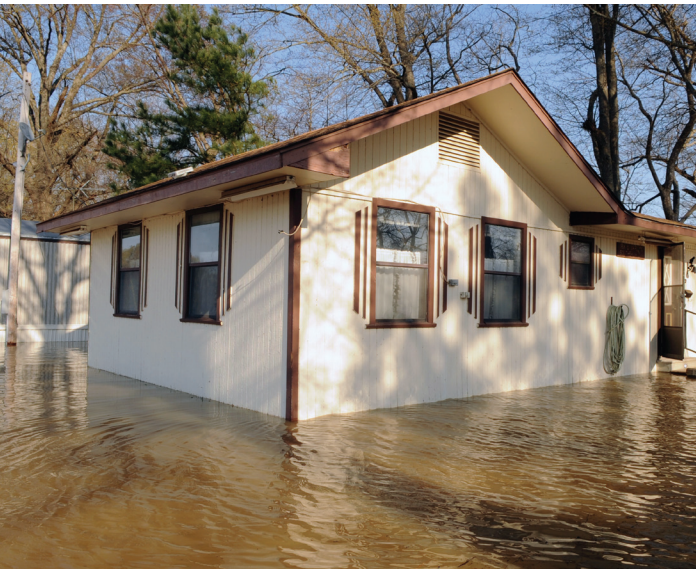
(ABOVE) DES ARC, AR, MARCH 25, 2008 -- THIS HOME IS SURROUNDED BY FLOOD WATER WHICH ROSE TO COVER THIS NEIGHBORHOOD AND COMMUNITY. JOCELYN AUGUSTINO/FEMA
