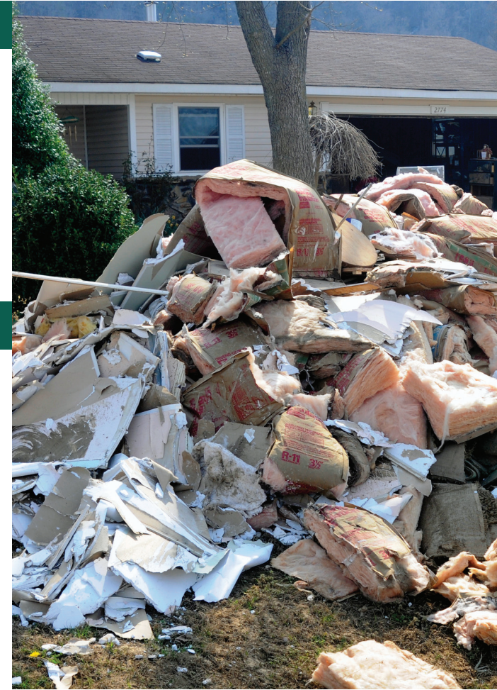
(ABOVE) NORFORK, AR, MARCH 26, 2008 -- PILES OF INSULATION AND CARPETING, STRIPPED FROM THE INTERIOR OF A HOME INUNDATED BY MORE THAN 36 INCHES OF WHITE RIVER FLOODWATERS, ARE STACKED AT THE CURB AWAITING REMOVAL FROM THE AREA. THIS HOME, ALONG WITH AN ESTIMATED 70 OTHERS IN BAXTER COUNTY, WERE AFFECTED BY A SEVERE WEATHER SYSTEM THAT SWEEPED ACROSS ARKANSAS IN MID-MARCH AND DUMPED AS MUCH AS 12 INCHES OF RAIN OVER A TWO DAY PERIOD IN SOME REGIONS. FEMA PHOTO BY WIN HENDERSON
